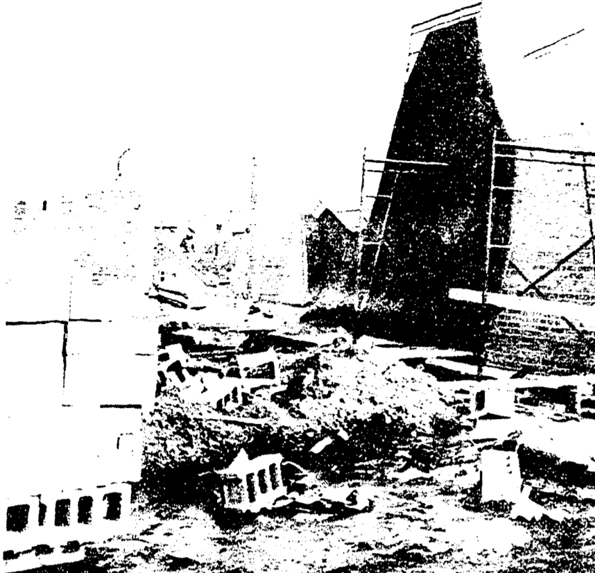
NORTHVILLE JUNIOR HIGH—With walls of the new Northville junior high school, located on Taft road, north of Eight Mile, rapidly nearing completion, construction officials predict that
