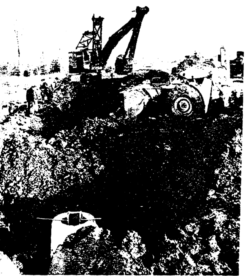
WIXOM SEWER CONSTRUCTION—Heavy machinery moving dirt is commonplace now in Wixom, ever since last week Wednesday when sewer construction began. Here, the first leg of the system is being laid in front of Holloway Construction company, the firm contracted for the job. That's a catch basin in the foreground.
