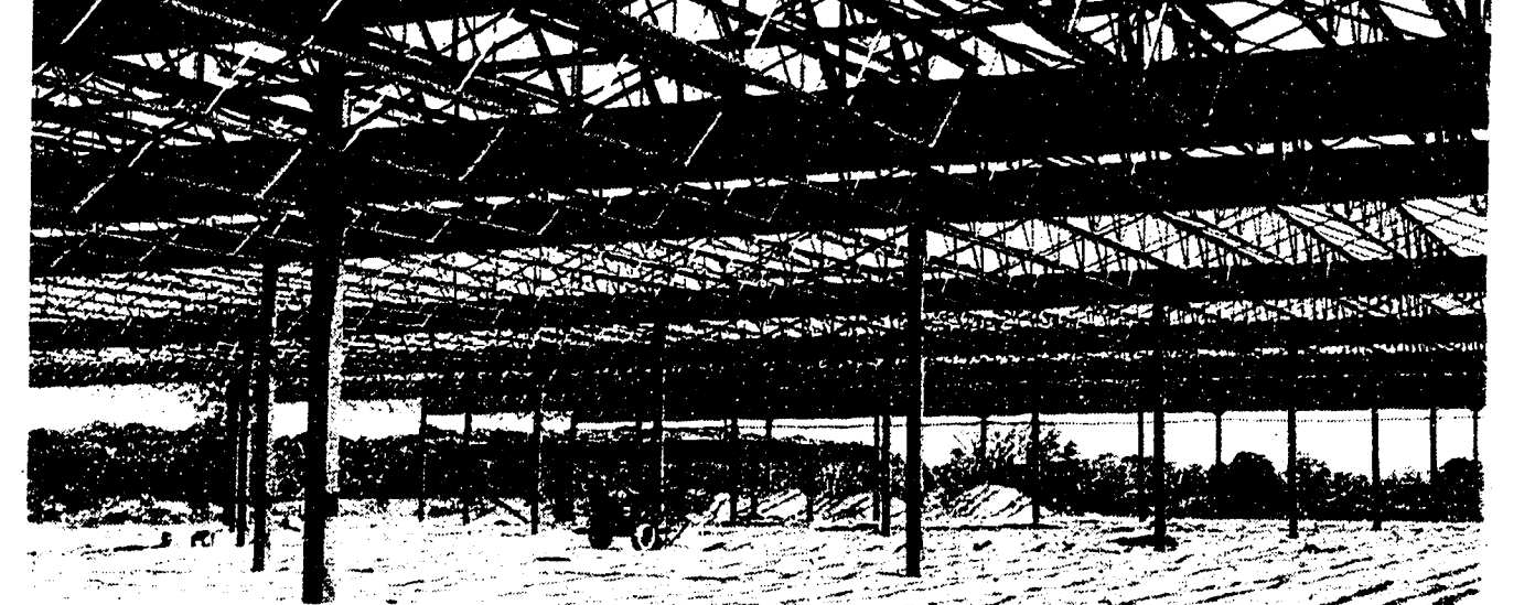
The ABC Photo building now under construction is Novi's biggest commercial project this year.
