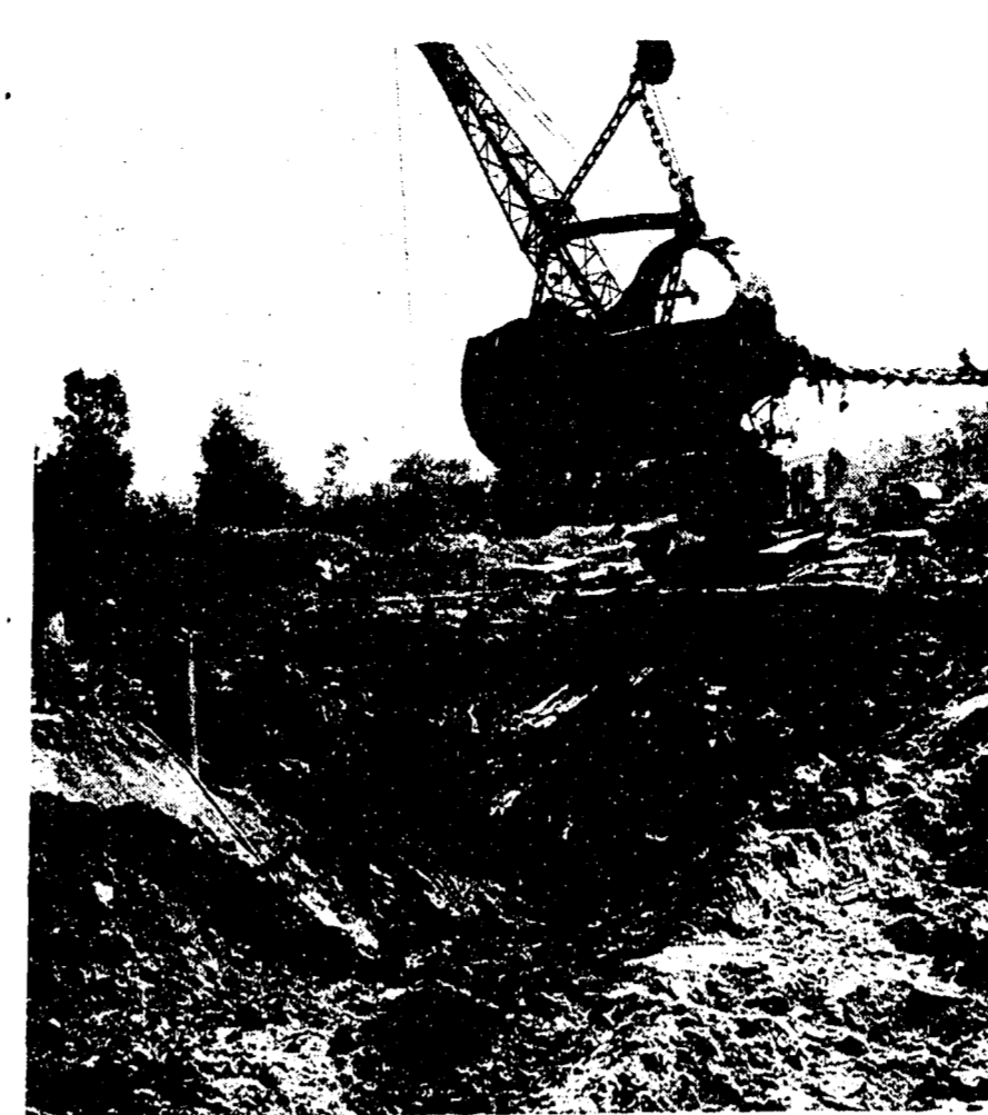
WATER BATTLE -Workmen installing Wixom sewers have had to battle water all the way. That's a well casing at the left, typical of the dozens that have been sunk to cope with the soggy locale.
