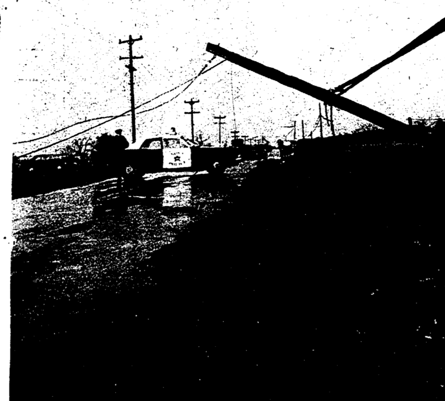
STORM DAMAGE—Slashing rain and wind, whipped up by tornado-like clouds, swept across the community Tuesday afternoon. One pole of the 'victims' was this utility pole on 10 Mile road. See story on Page 5-A.
