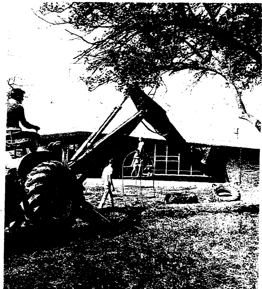
PLAYGROUND UNDERWAY - It isn't much yet, just a few holes, giant tires and large tiles. But when the playground is finished, kindergartners at Orchard Hills Elementary School will have their own fun area adjacent to an apple orchard just outside their classroom. The playground is one of the projects of the Orchard Hills Booster Club formed late last year.
