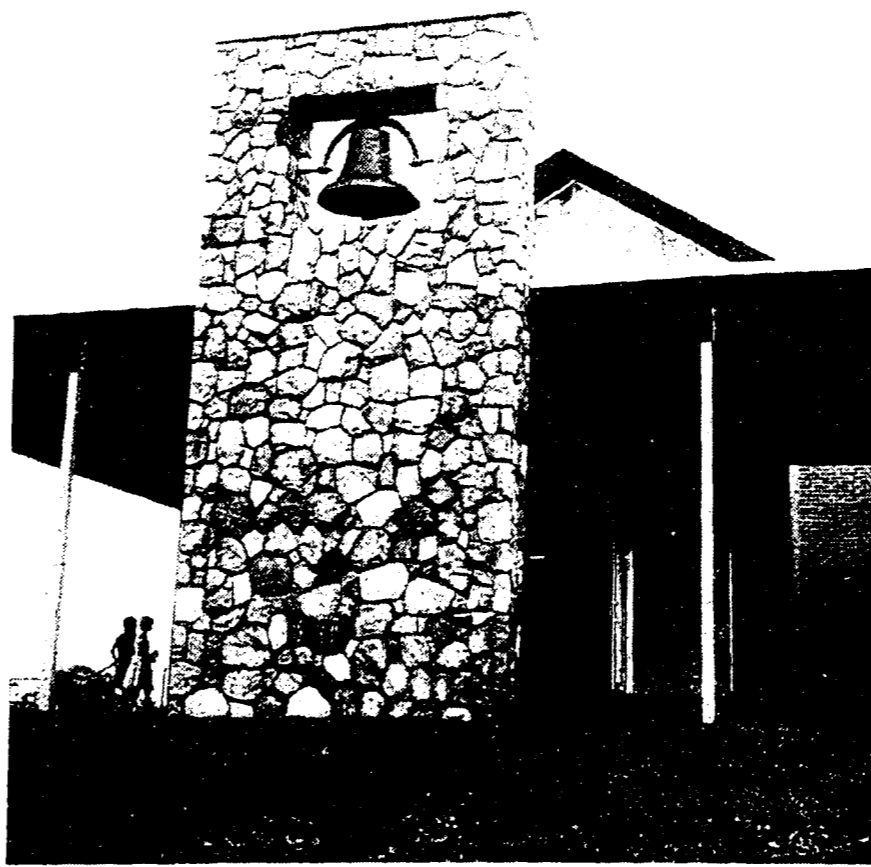
NEW BELL TOWER—housing the old church bell, which dates back to 1865 at the Wixom First Baptist Church, was a feature of the dedication Sunday of the new educational addition. (See related pictures on page 12-A).
