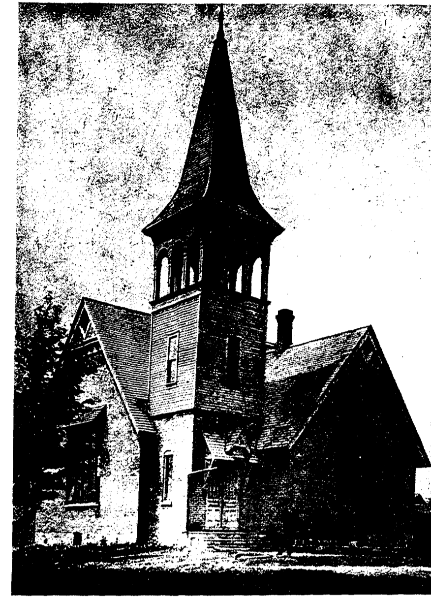
This was the way the church looked before the spire was chopped off.
