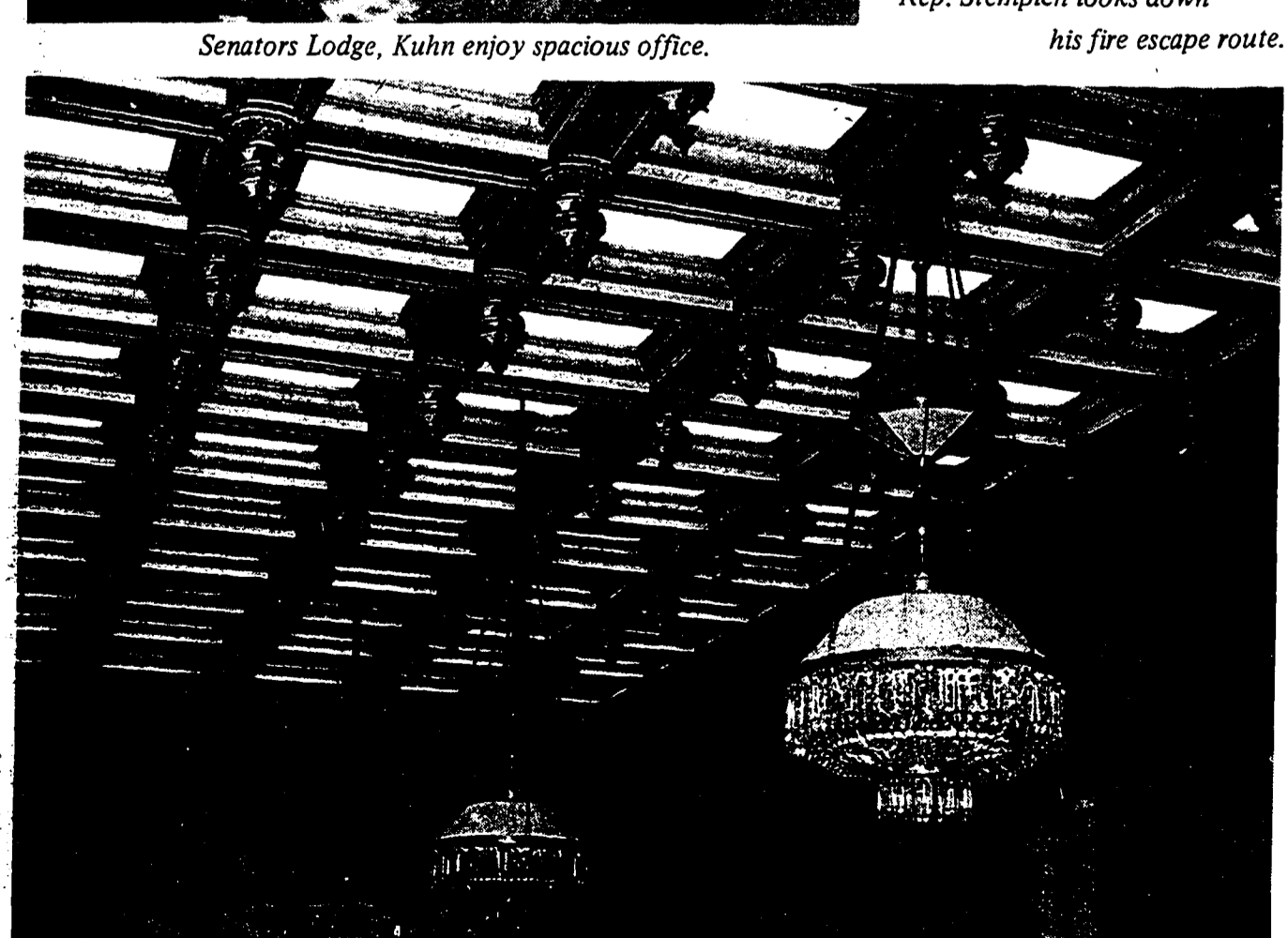
It's beautiful but leaking roof turns chandeliers into crackling firworks.
