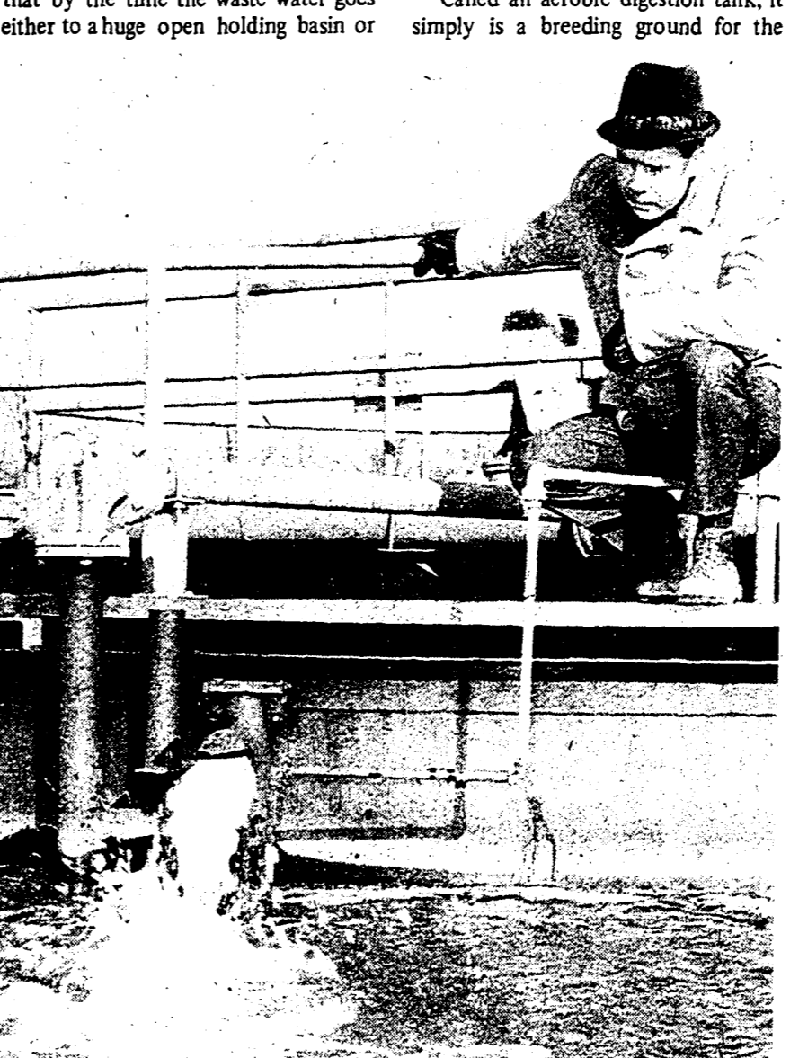
BUG TANK - Project Engineer John Albrecht inspects Wixom's new sewer disposal system where microscopic bugs help keep the city clean.
