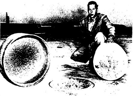
DIAMOND BIT - Shown here (left) is the giant 24-inch diamond bit that recently gained national attention for drilling holes in concrete runways at Chicago's O'Hare Airport. At right is a 20-inch concrete core and a semi-completed hole is shown at the center.
