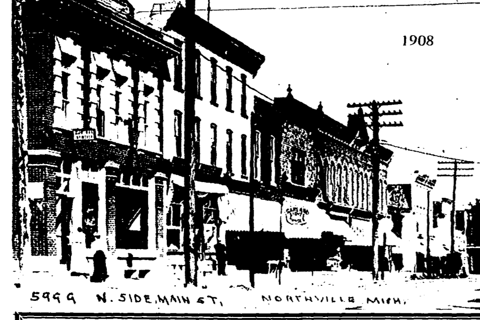
BUILT IN 1870 - This old building, which featured an overhanging "balcony" on Main Street, was razed in 1958 to make way for the municipal parking lot on the north side of the street, west of The Record building. At the time it was razed Frank Hill had been operating a real estate business there. Earlier it was the "Hill Meat Market."
