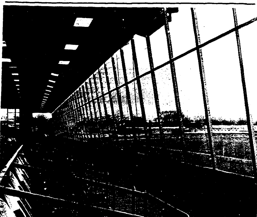
WINTERIZED - Northville Downs grandstand has been completely enclosed in glass to permit summer temperatures for winter racing that begins Monday.
