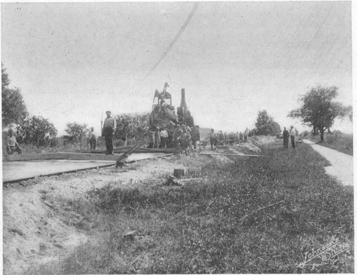
Paving outfit on the Rochester Road.
