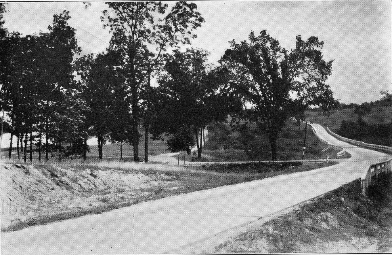
Long Lake Road (over new right of way)
