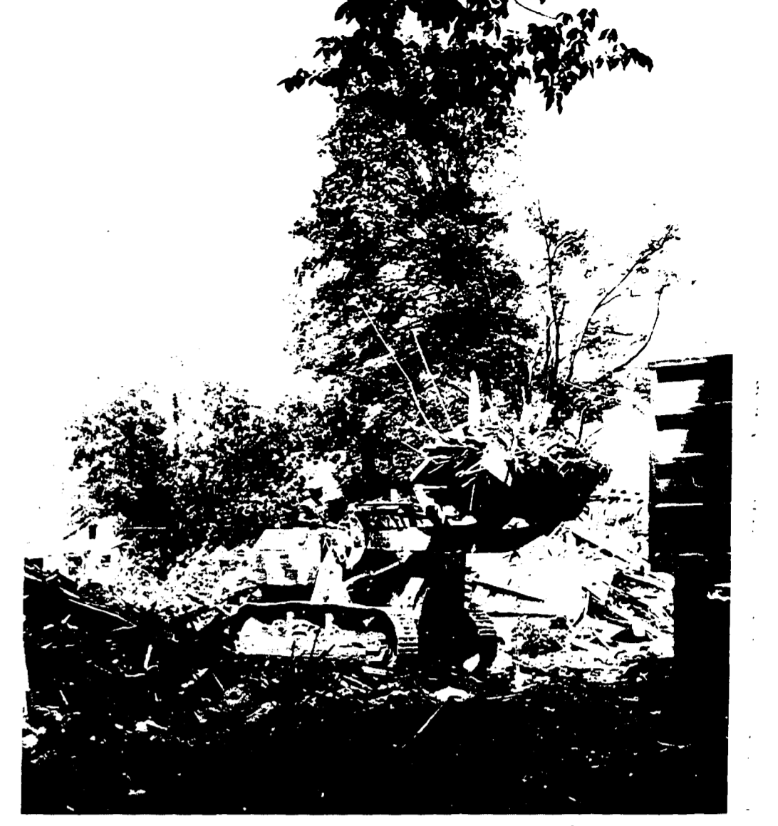
Bulldozer Prepares Northville Square Development Site
