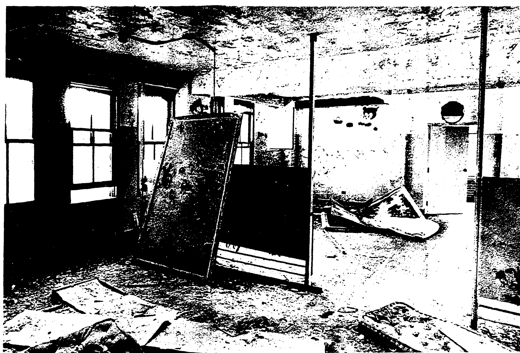
Everywhere you look—inside and out—vandalism and abusive weather has reduced Maybury buildings to just a ghost of what once was one of the world's most widely acclaimed TB Sanatoriums. The buildings are to be razed soon to make way for the first state park in Wayne County.
