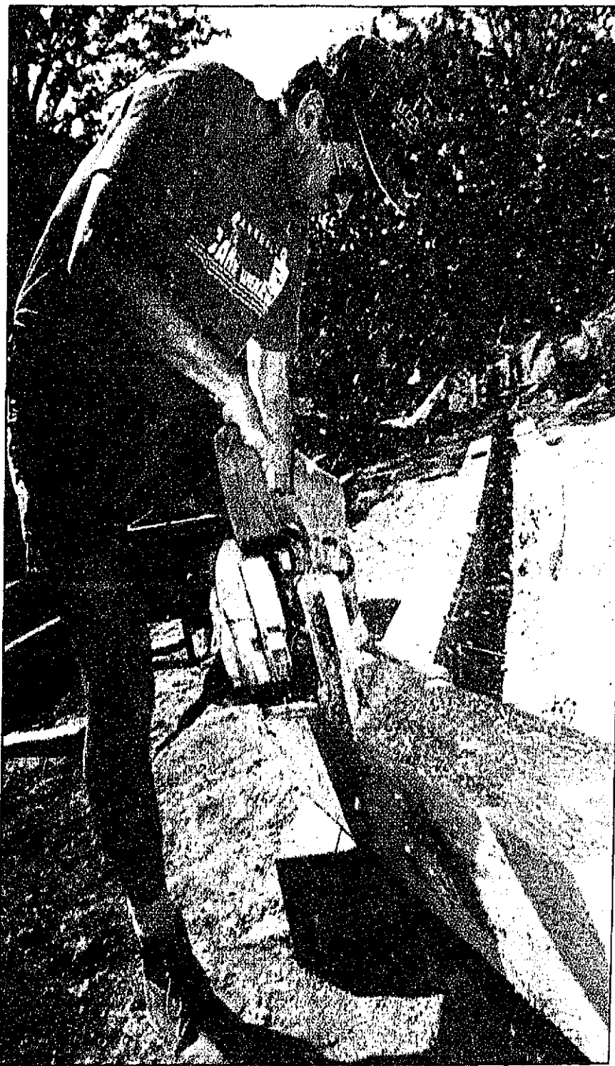
Volunteer Ted Mech wields a chainsaw Saturday morning, cutting railroad ties for the retaining wall.
