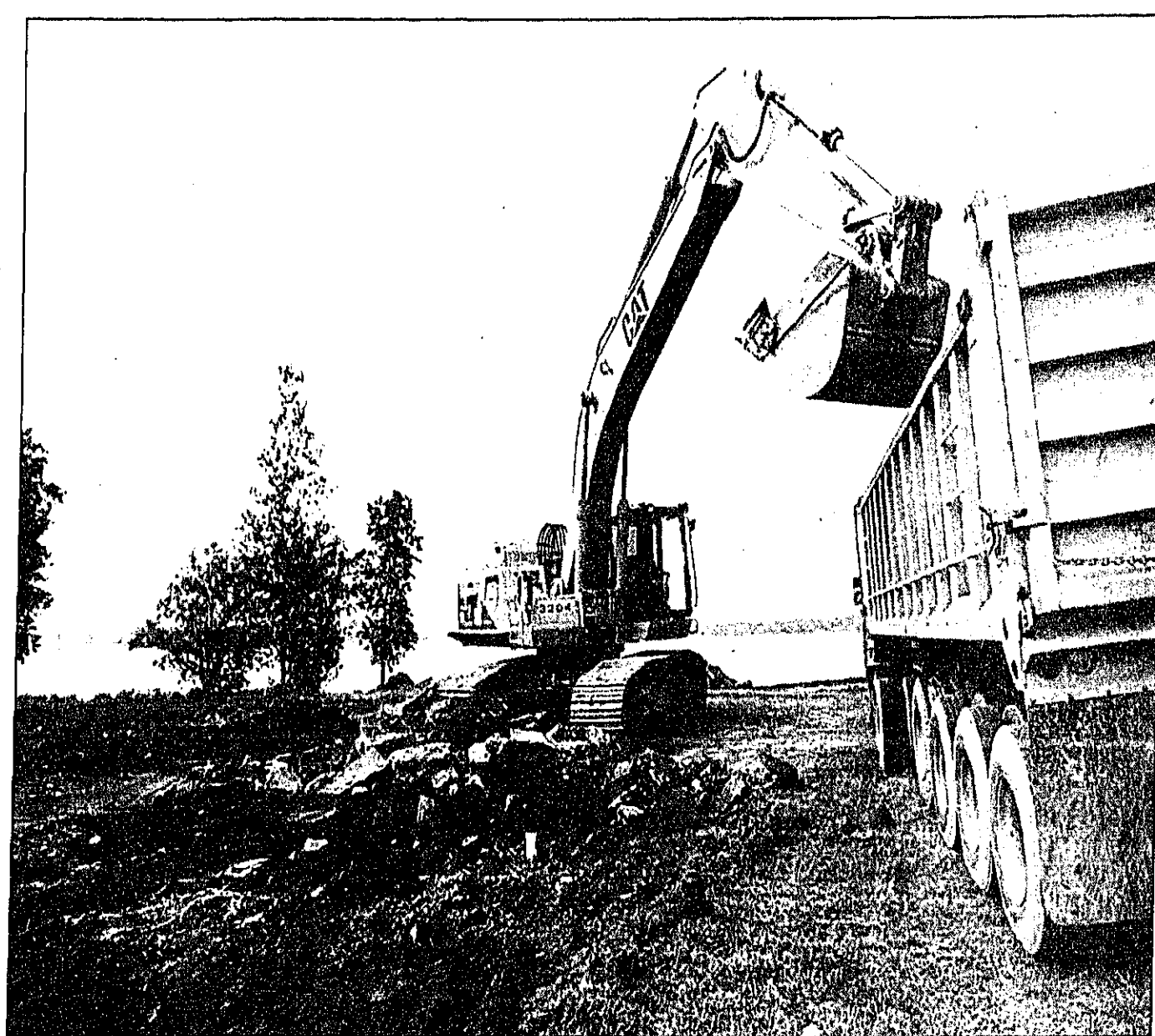
Workers rip up an old roadways at the site of the old Walled Lake casino and amusement park.
