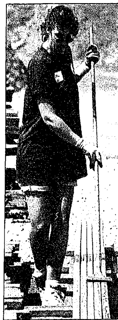
Volunteer Val Blue varnishes rails to prepare them for installation.
