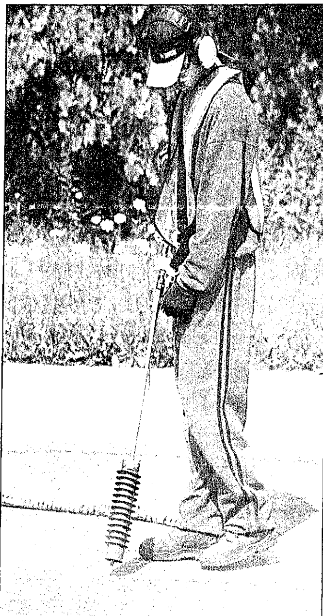
Crew members like Marc Tolsdorf go through one pair of work boots each summer because of the intense heat of both the torch and applicator used in the hot patch road repair. Right: Bob West uses the torch to remove old tar, debris, and moisture from cracks that have formed in the road surface.
