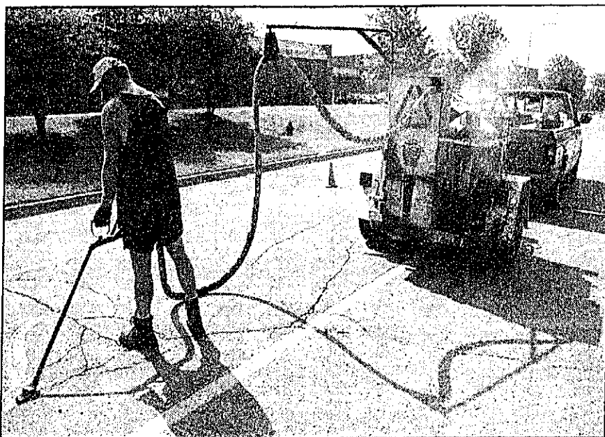
Left: Bob West is required to wear a protective vest and boots; safety vest, glasses and ear muffs; and long sleeve shirt and pants when working the torch which has an exhaust gas of 2,200 degrees. Above: Marc Tolsdorf works the applicator on a road behind Novi's West Oaks Mall to apply the rubberized compound which is 370 degrees.
