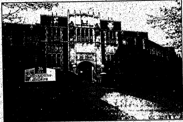
Child care plan: Oakland County officials may renovate the former Children's Village into a day-care center for county employees.
