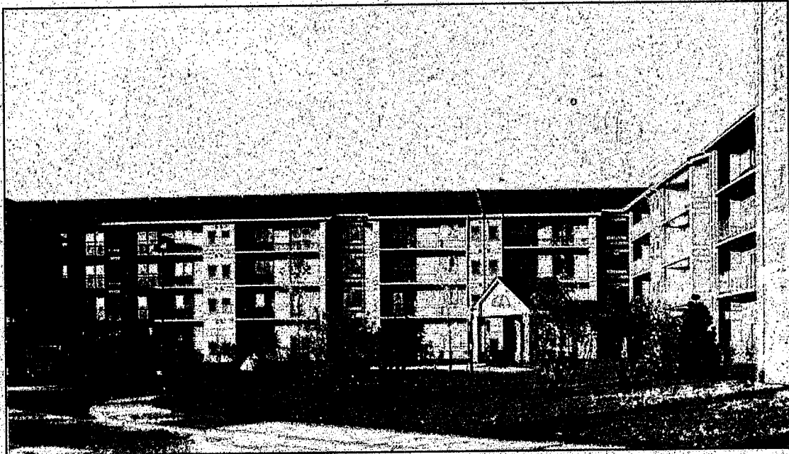
Mid-rise apartments: Concrete, split-faced, dyed blocks present an attractive appearance at Eagle Pond Heights in Walled Lake.
