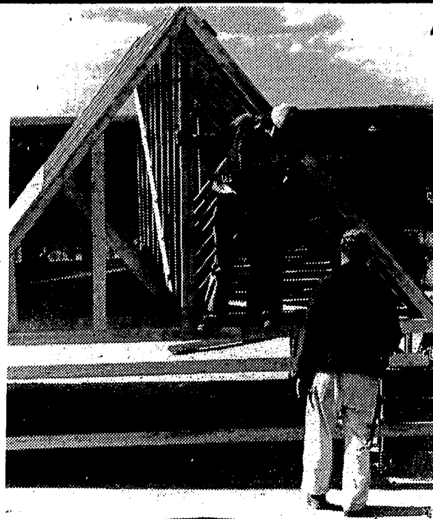
A-frame housings are made to cover the upper terminals of the lifts eliminating the need for time-consuming snow removal later in the season.
