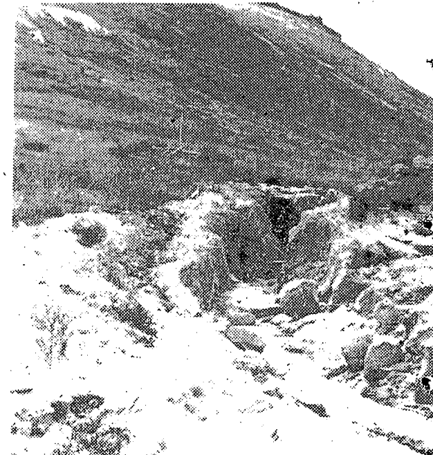
A-frame housings are made to cover the upper terminals of the lifts eliminating the need for time-consuming snow removal later in the season.
