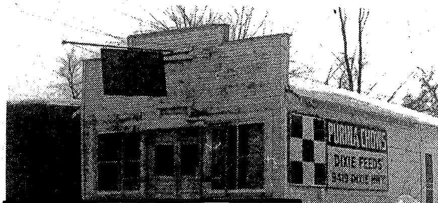
The Dixie Feeds Store [c. 1870?] is an example of a simple false-front building. In other words, the facade does not correspond to the actual roof line, but, instead, rises above it. This convention was often used to increase the visual impact from the street level. There were many such buildings in downtown Clarkston into the 20th century.
