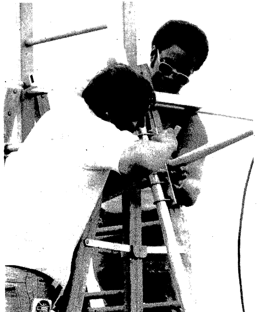
John Van Putten [Davisburg] and Bob Patton [Pontiac] attach a beam antenna which receives world-wide radio signals.
