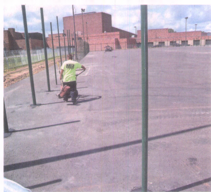
Resurfacing continues Aug. 3 on the tennis courts at Novi High School. The courts were closed in mid-May and should be open and ready for players by the end of August. Courts will feature new fencing, nets and playing surfaces.
