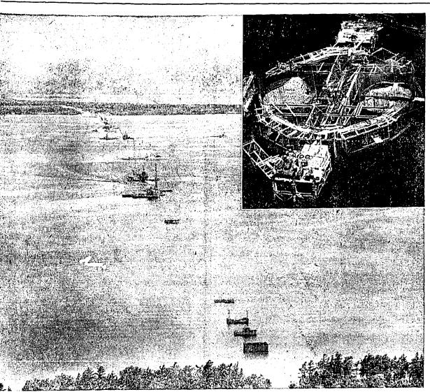
foundations clearly show the route corner shows main tower foundation. The two 38 ft. in across the Straits. North from Mackinaw City, aerial photo diameter towers are being constructed on the caisson shows all but six foundations on the south side and all the foundation, 116'ft. in diameter. The latter will be cut off foundations on the north side, including the causeway in at 8 ft. below water and the 527 ft. high tower will rest on
