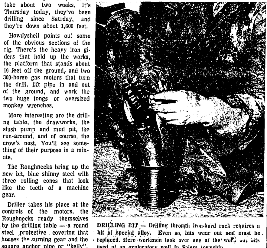
DRILLING BIT — Drilling through iron-hard rock requires a bit of special alloy. Even so, bits wear out and must be replaced. Here workers look over one of the bits, as bits used at an exploratory well in Salem township.
