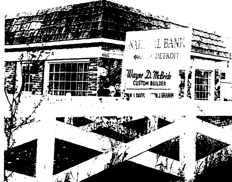
NEW BANK — National Bank of Detroit opened two branch offices here last week in temporary quarters. This one is located on Seven Mile Road, east of Northville Road. The other, in Novi, is located on Eight Mile, west of Haggerty.
